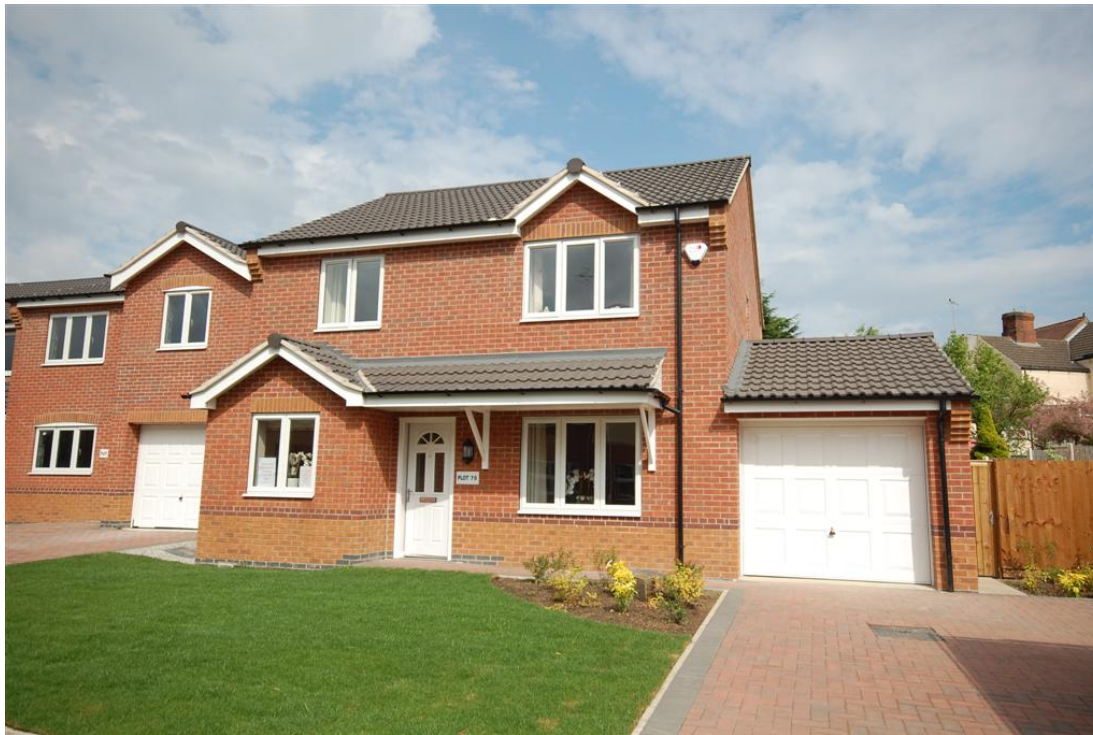
Picture shows a typical BGA1 – Baltimore
